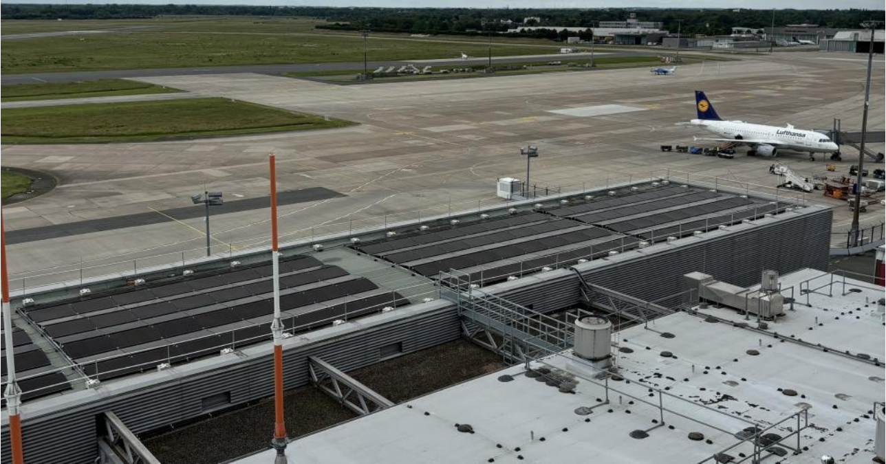
A photovoltaic system on the roof of the Bremen control centre has been supplying the DFS branch with solar power since 2023. (Photo: DFS)
