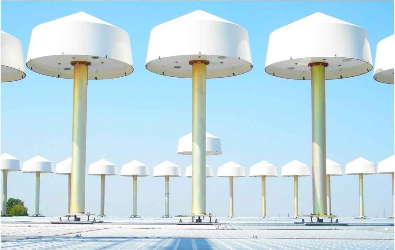
The protection zones around Doppler omnidirectional radio beacons, such as the DVOR Ottersberg, have been reduced from 15 to 7 kilometres. (Photo: DFS)
